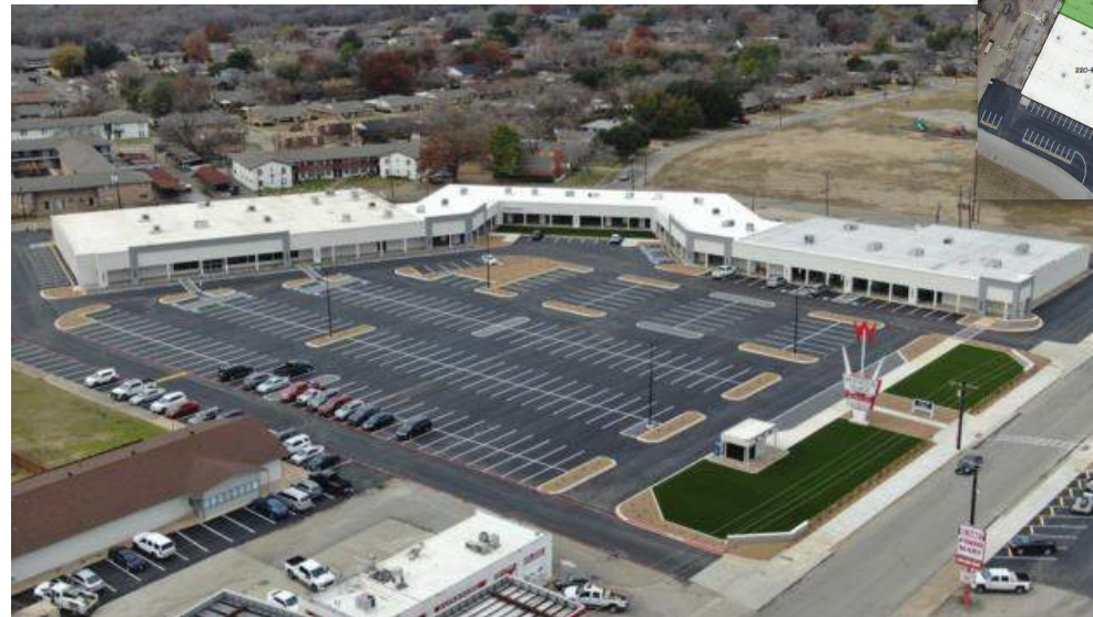
After (Drone Photo)
